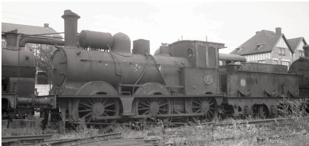
Former LNWR DX Special 3287, later MT 18, pictured in the ownership of SNCB/NMBS yet retaining the identity of MT 18" until its withdrawal. The locomotive is pictured at St Niklaas depot 10/08/1948. The Westinghouse brake apparatus can be seen on top of the boiler. Joop Quanjer, Collection NMBS/SNCB – Train World Heritage
